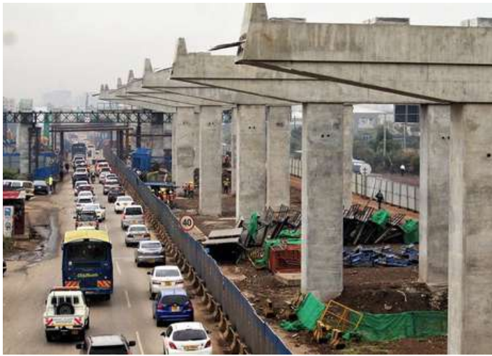
Construction of the Nairobi Expressway
